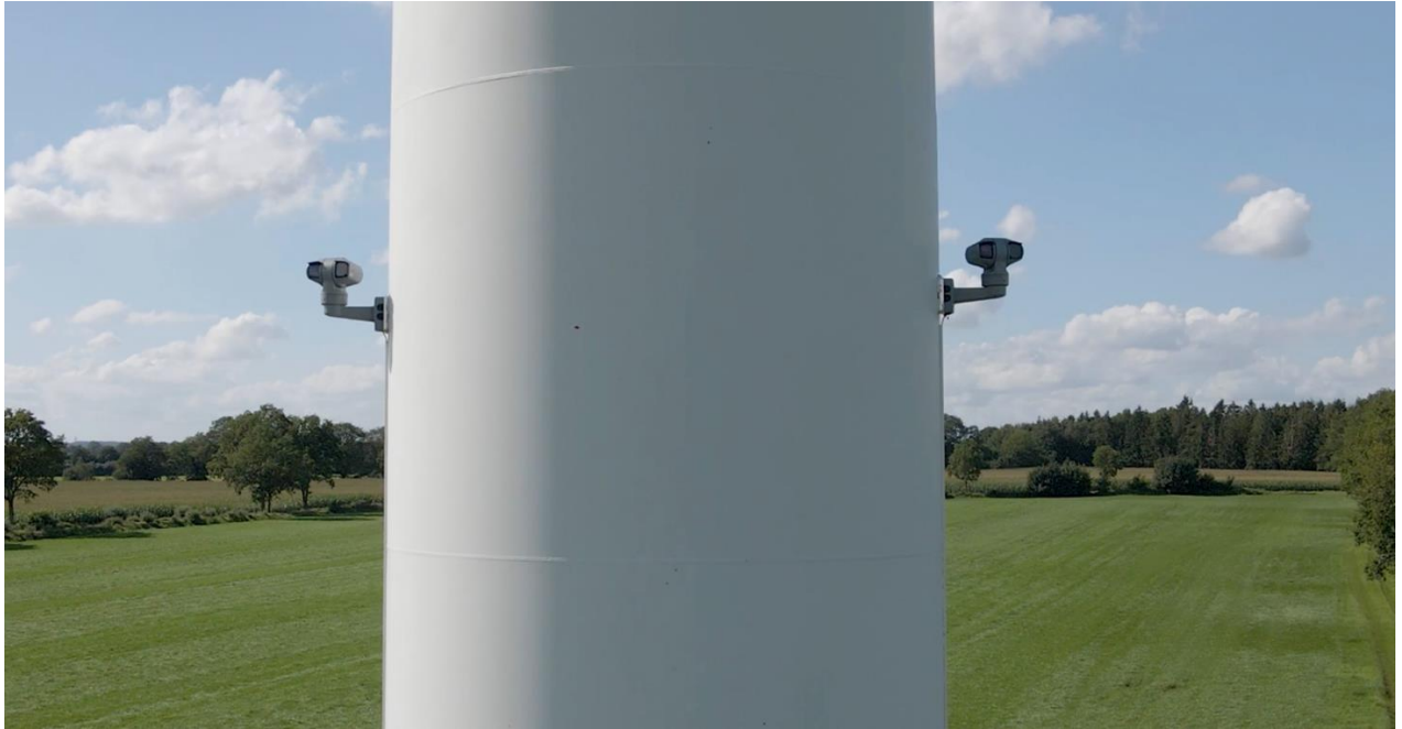
Figure 6: Camera systems at the tower of the Gnutz-Timmaspe wind turbine.
